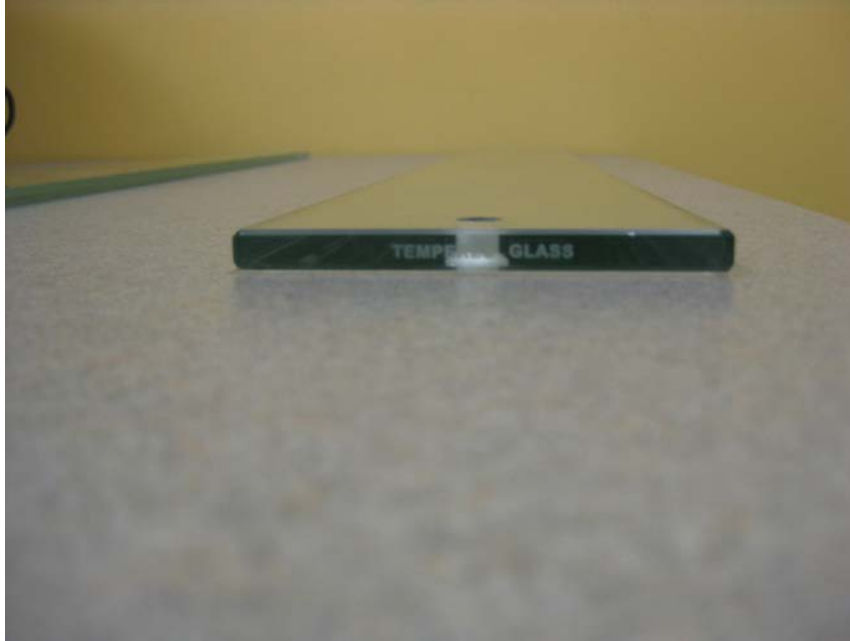
Photo No. 12 Permanent Marking on One End of Glass Balustrade – TEMPERED GLASS
