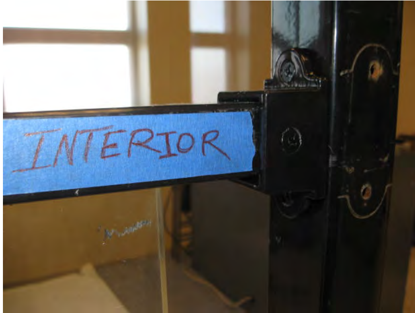
Photo No. 10 Typical Rail Bracket Connection
