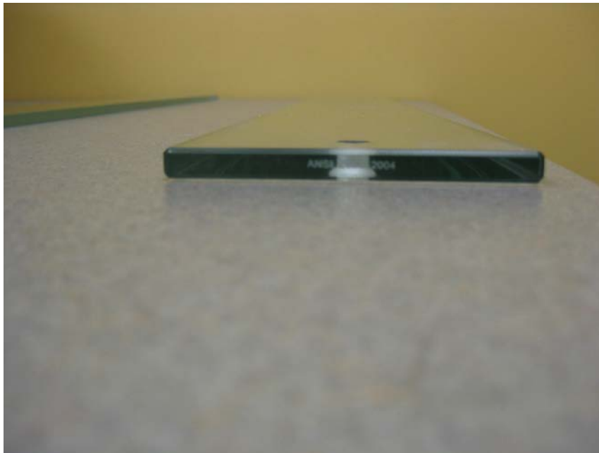
Photo No. 11 Permanent Marking on One End of Glass Balustrade – ANSI Z97.1-2004
