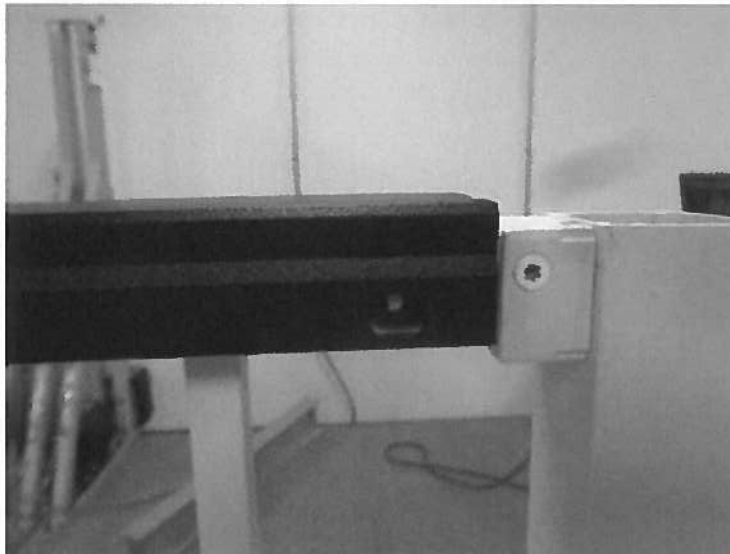
Photo No. 8 Rail-to-Post Connection
